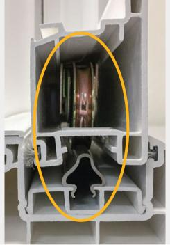
Door rollers glide over a durable, one-piece stainless steel track with effortless operation for a lifetime.
